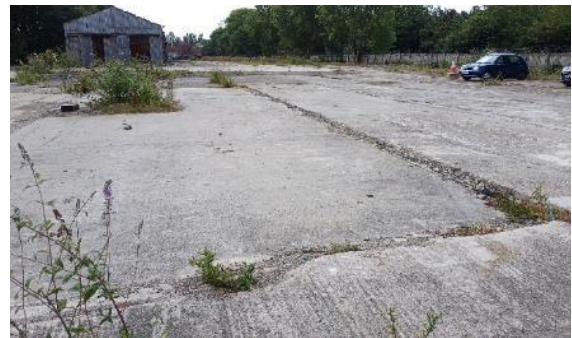
Photograph 2: Hardstanding with scattered buddleia scrub (06.08.2025).
