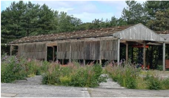
Photograph 3: Building (B4) on-site (06.08.2025).
