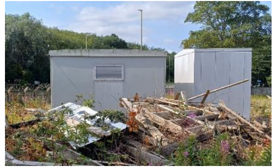
Photograph 4: Building (B7) on-site (06.08.2025).
